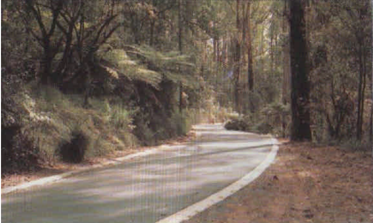
Sherbrooke Road Kallista was reconstructed in harmony with the surroundings, following concern for the environment expressed by local residents.
